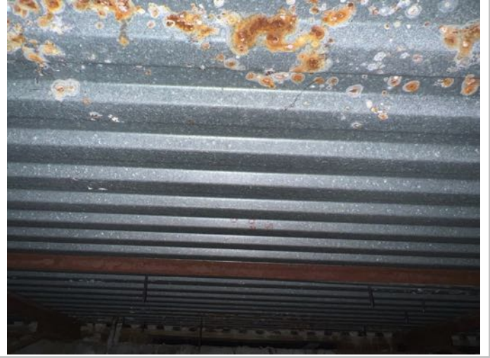
corrugated concrete deck form
